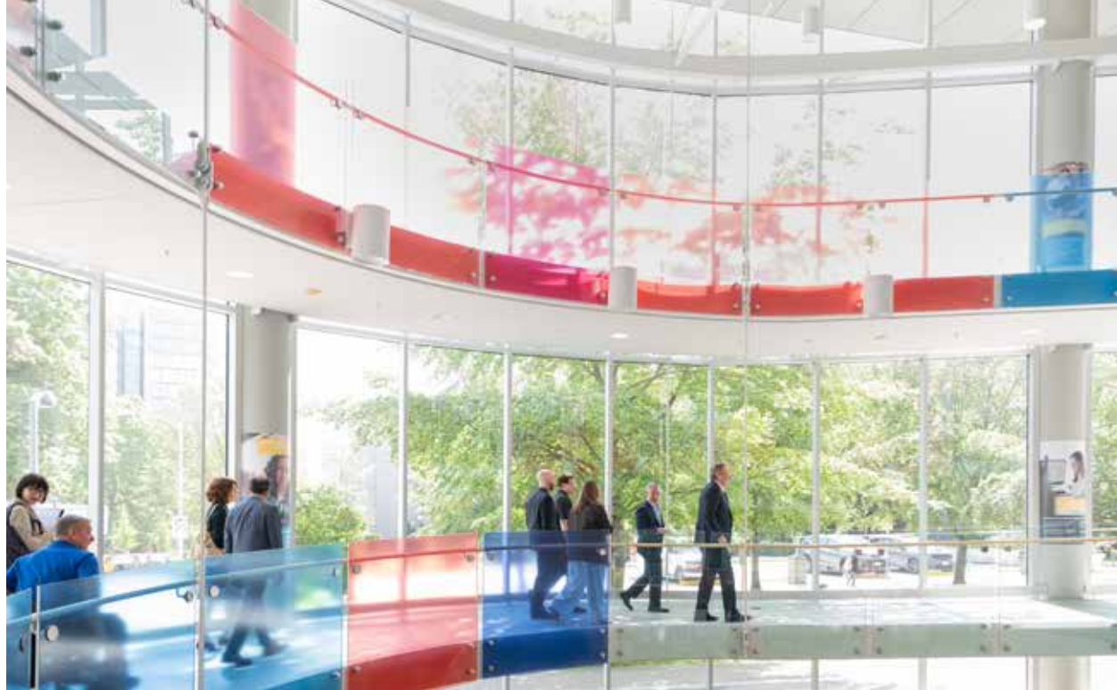
A ramp with a gentle incline winds around the atrium at the Blusson Spinal Cord Centre, giving wheelchair users an alternative to the elevators. Photo: Martin Dee
